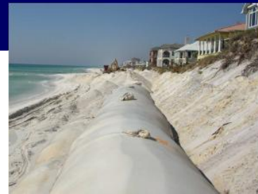
Marine Containment Structure
